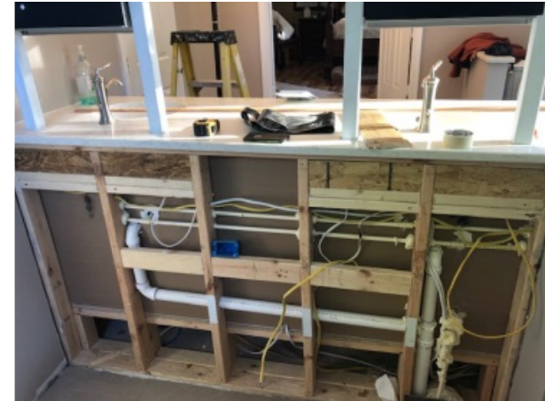
Hidden wiring and pipes; reinforced supports
