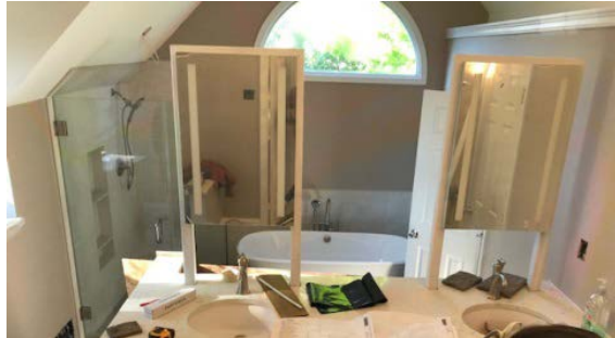
Steel tubes to “float” mirrors meant exact cuts in quartz countertop to fit tubes and sinks.
